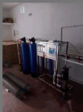
SODA PLANT INSTALLATION SERVICE
