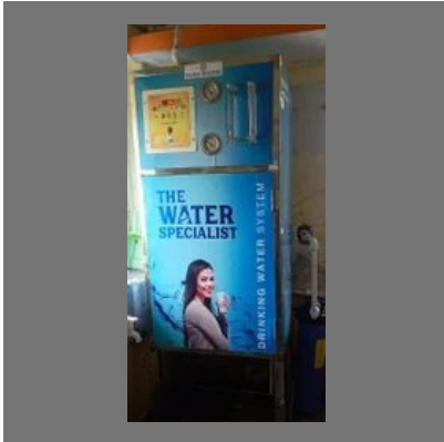
150 Lph Ro System
